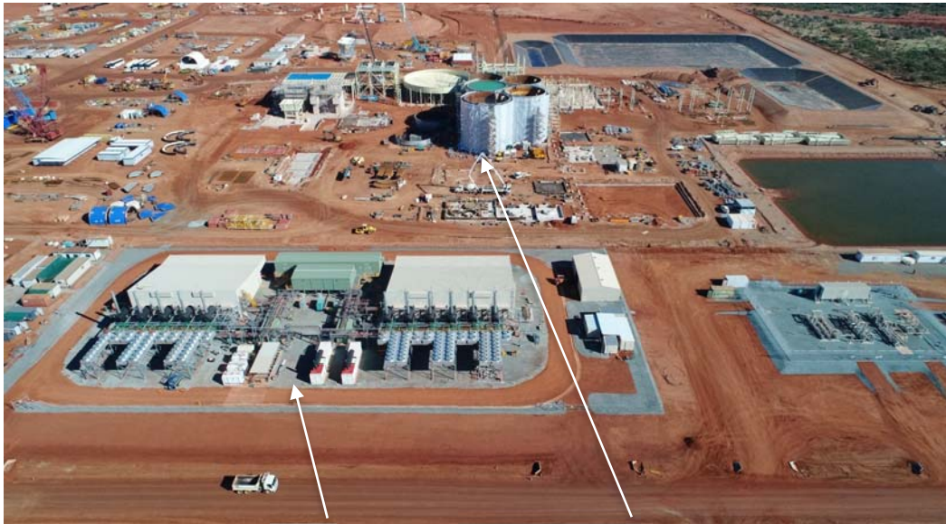
Aerial view of Power Station (foreground), Process Plant (background)
